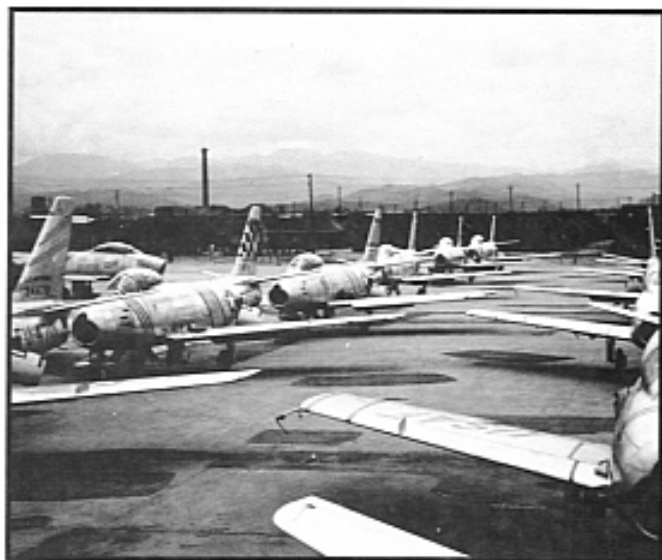
The Tsuiki REMCO Parking ramp in 1953.
