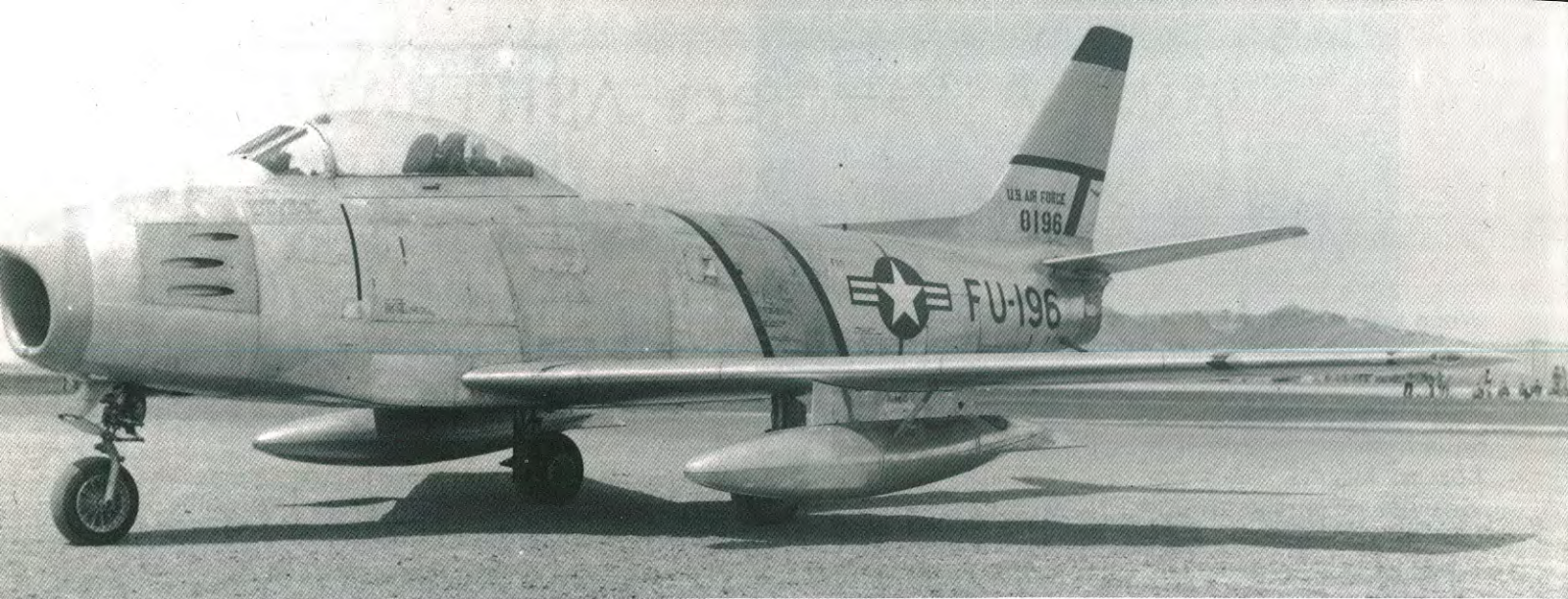
The first RF-86A ASHTRAY on rollout from the Tachikawa modification hangers. The ASHTRAY airplanes had two cameras in the bulged lower fuselage, with a dicing camera mounted in the upper nose. Note they still had paint schemes similar to the 4th FIG F-86s. (USAFM)
