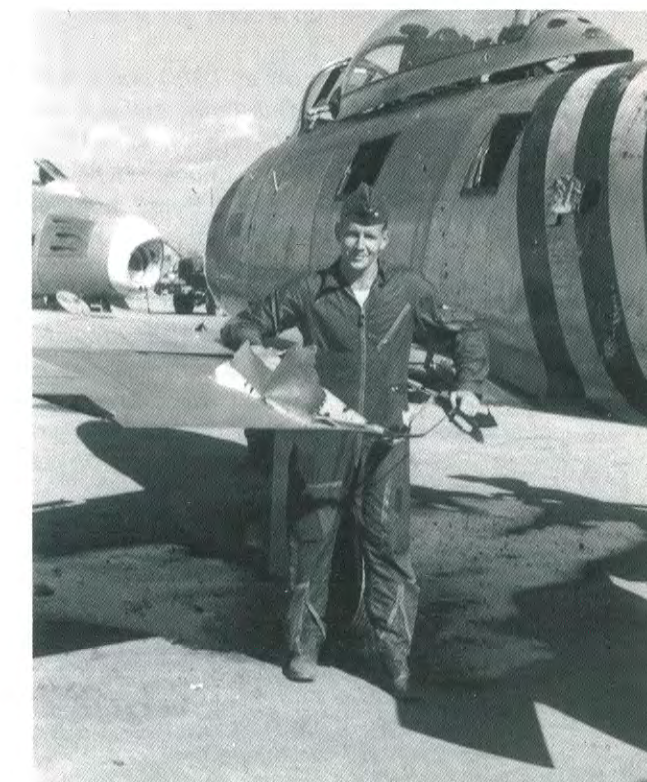
Lt Chuck Loyd stands in the hole where a MiG 37mm cannon shell struck his flap. The damage looks extensive, but this Sabre would fly and fight again. (Robert Makinney)
