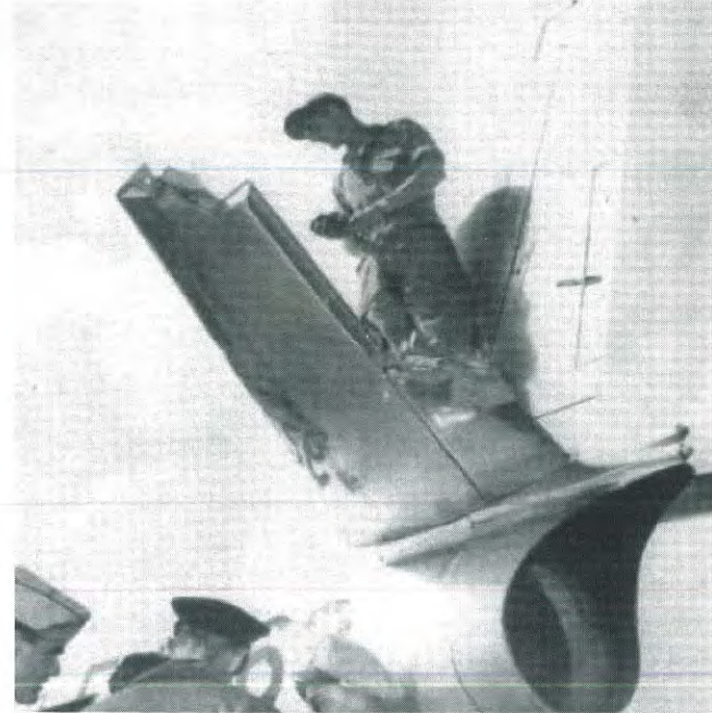
Two photos showing the damage to Bruce Cunningham's elevators. The high sustained Gs of the race broke off both elevators during the final turn of the Thompson Race. This airplane now resides in the MAPS Museum at the Akron-Canton Airport, Ohio. (credit USAF)
