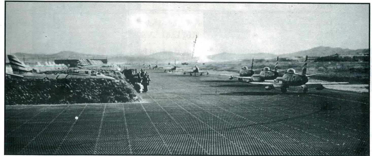
A gaggle of 35th FBS F-86Fs taxi down the PSP ramp to the runway at K-13 in 1955. Sandbag revetments were built between every aircraft due to possible night attacks by sappers or North Korean raiders. (credit - Ozzie Neidermann)
