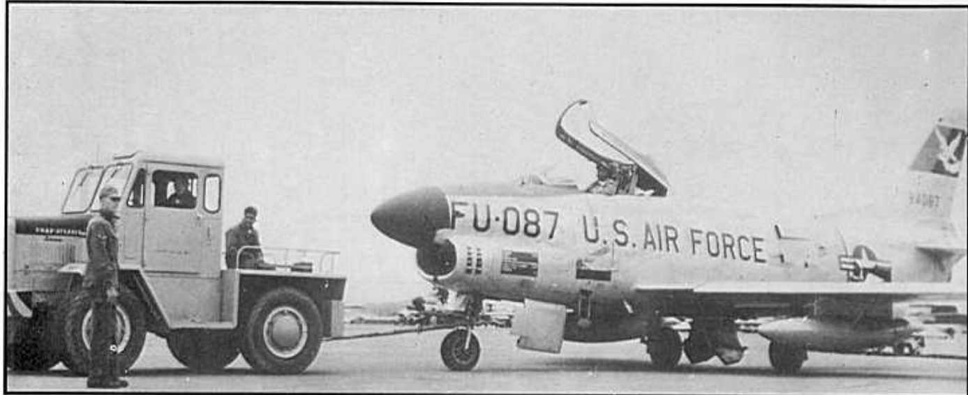
An F-86L-60 assigned to the 330th FIS at Stewart AFB, NY in 1957. The additional engine cooling scoops used on the F-86L can be seen just aft of the fuselage letters. The 330th FIS took delivery of their first Ls in December 1957. (credit - Marty Isham collection)
