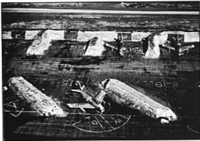
36th FBS revetments at Suwon in the Summer of 1953. The revetments were constructed from old fuel drums with sand bag walls. (credit - R.C. Hyatt)
