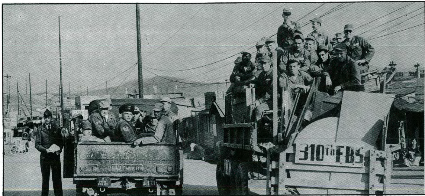
Members of the 310th FBS supported the Sung Yook Orphanage near Osan in 1957. This truckload of 310th personnel are taking scrap wood to Sung Yook to be used for firewood and patching the building against the December cold. (credit - Floyd Montgomery)
